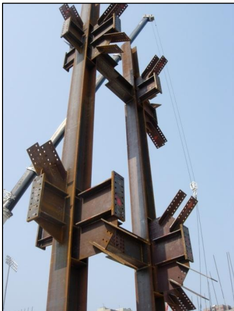
Figure 6: Connection construction photo
